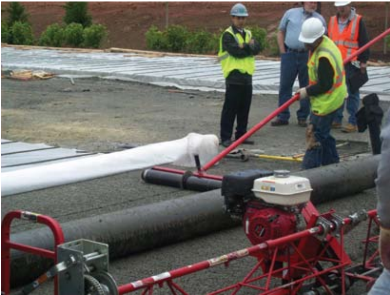
The pervious concrete being rolled and cut in a construction joint
