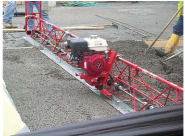
The pervious concrete being leveled with a vibratory screed
