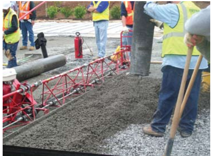
The pervious concrete being placed
